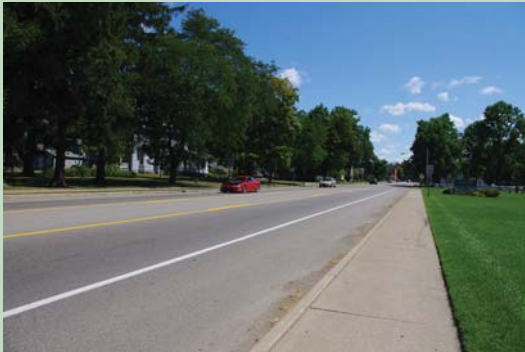
This section of M-139 is designed for cars and not people. Note the lack of buildings built near the street, high traffic speeds, and no buffer between the sidewalk and the road.
