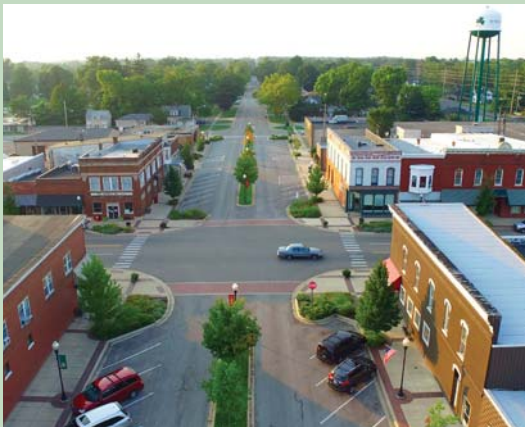
This section of Main Street (near Ferry Street) is designed for everyone including pedestrians due to extensive landscaping, street lights, bulb-outs, well-marked crosswalks, and buildings constructed up to and facing the sidewalk.
